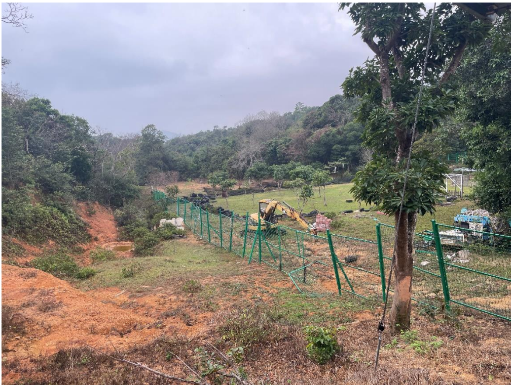
Photo H General view of southern end of the Site, looking west
